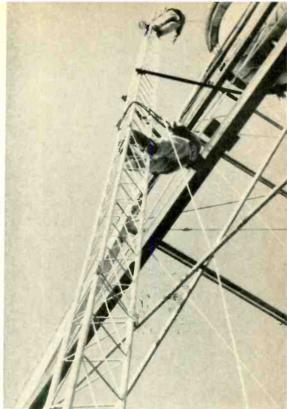
Valley Vision system in Jackson, Cal. utilizes 105' tower alongside abandoned water tank once used to supply famous Argonaut gold mine.
